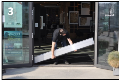
Lower beam (with bottom seal) first. NB. when the beam is mounted, the bottom seal, should sit in the groove throughout the length of the beam
