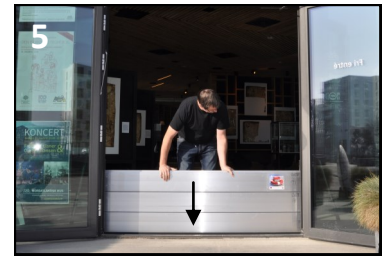
The beams must be pressed together and down towards the floor so that the bottom seal can absorb unevenness in the floor
